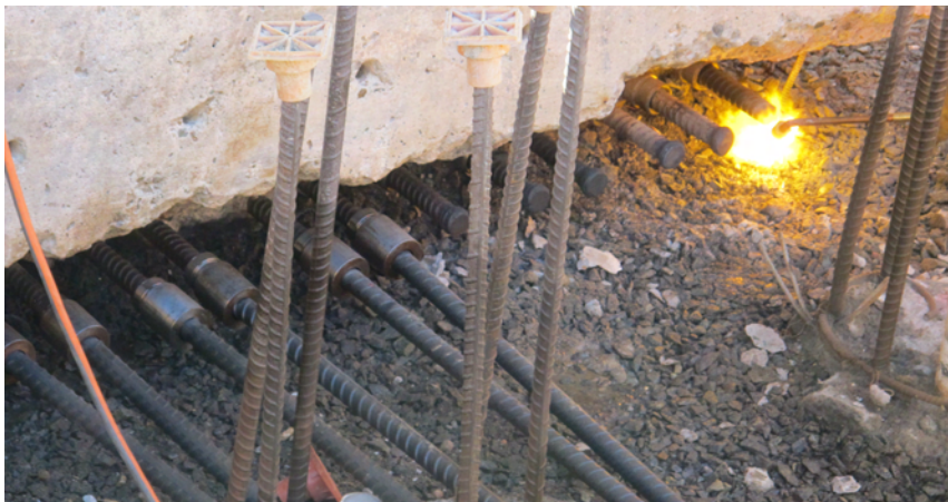
Heating the end of the bar before forging the upset head
