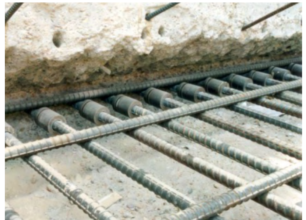
Completed foundation connection
