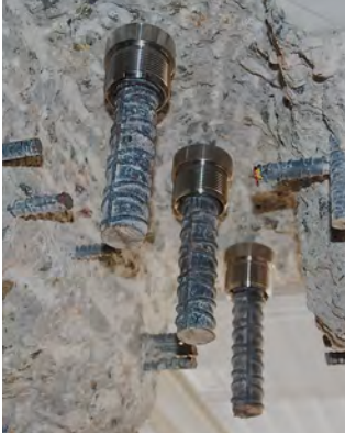
Before and after installation of upset heads on #11 Rebar
