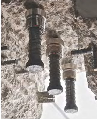
Before and after installation of upset heads on #11 Rebar
