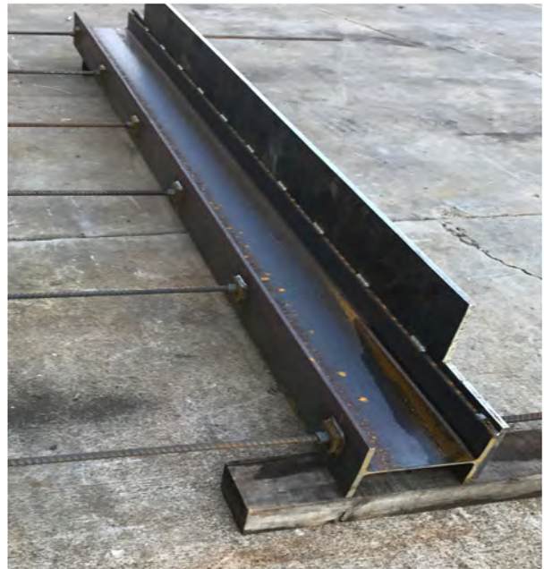
Dowels at Steel Beam/Lintel
