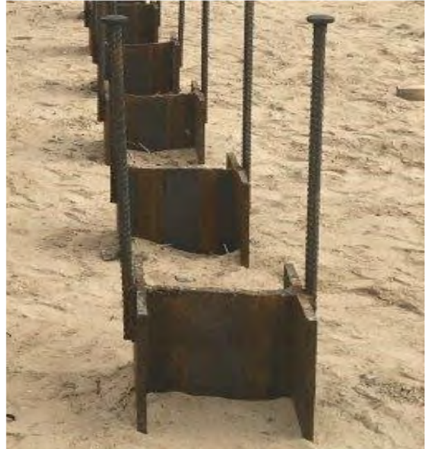
Welded Pile Anchorage
