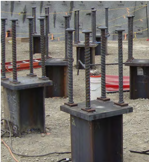
Pile Anchorage (w/ head plate)
