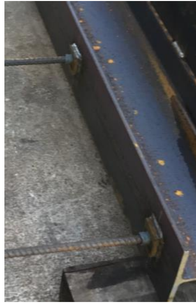
Dowels at steel beam/lintel
