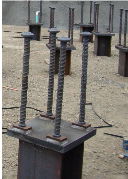
Pile anchorage (with head plate)
