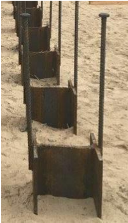
Pile anchorage (welded to pile)
